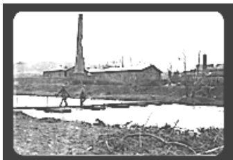
C Company's footbridge across the Roer River – March 1945
