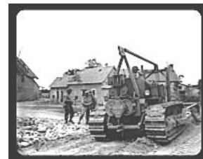
One of 299 th Engineer Battalion's eight bulldozers that landed at Omaha Beach
