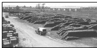
Curtis Bay Storage Activity
